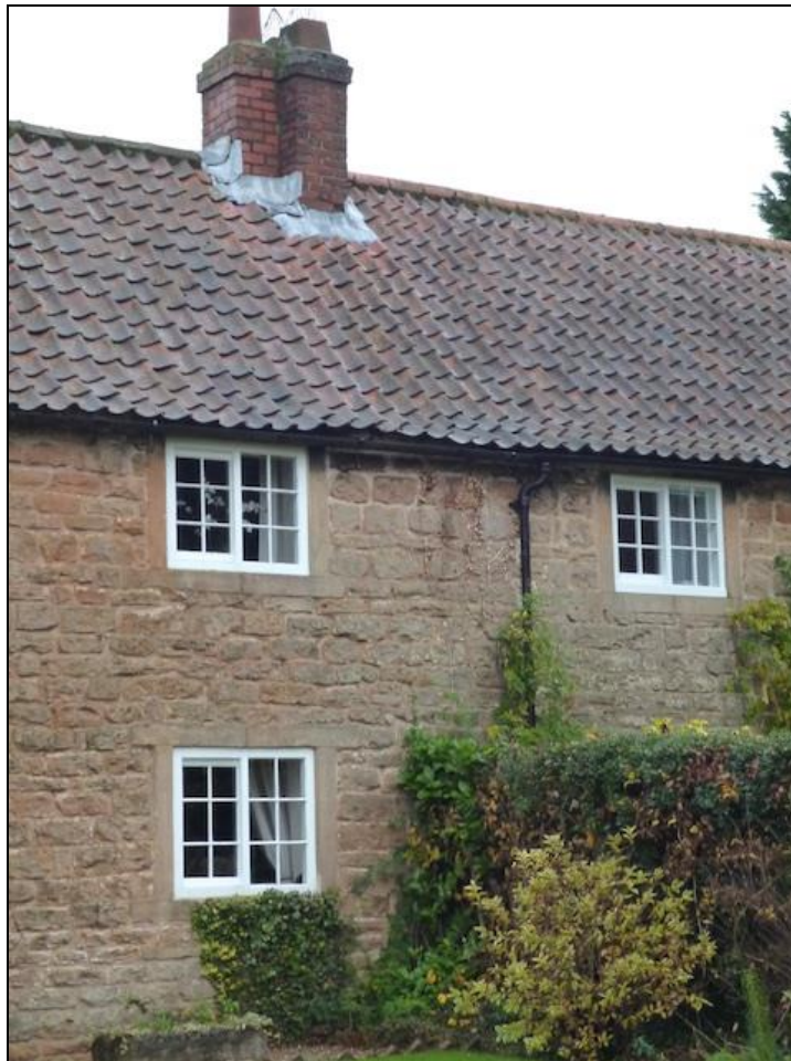
Photo 21: Details of local construction methods and materials, at nos. 67-73, Main Street, illustrate the use of local magnesian limestone with a pantile roofs and Yorkshire (horizontal) sliding sash windows
